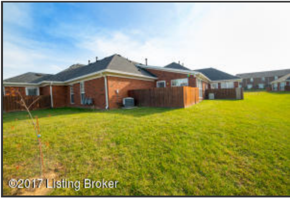
Grounds and exterior are well maintained
