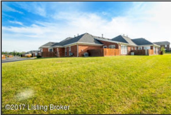
Grounds and exterior are well maintained
