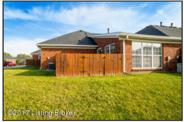
Grounds and exterior are well maintained
