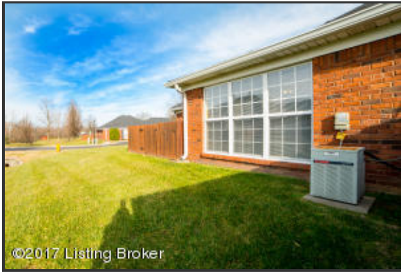
Grounds and exterior are well maintained
