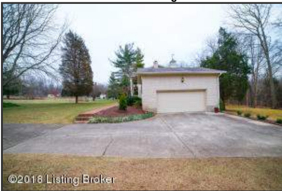
The extra-wide driveway approaches the roomy two-car garage and offers space for additional guest parking
