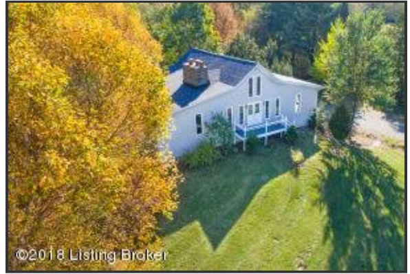
Roof Just Six Years Old
