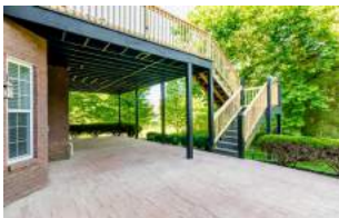
Lower Level Patio
