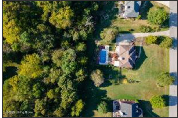
The roof is less than 10 years old
