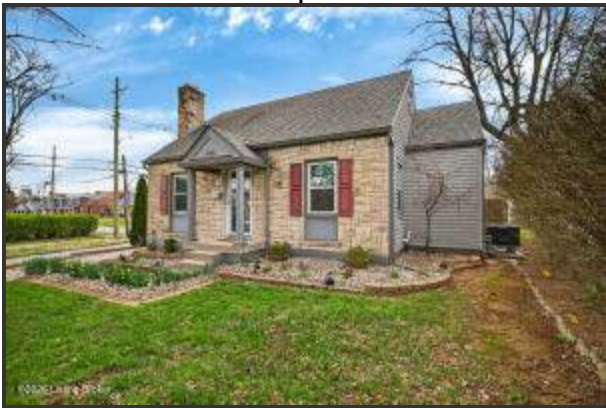
New roof installed 2018 with leaf system
