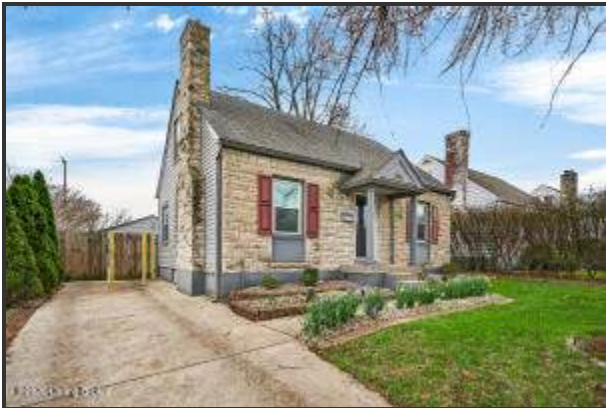
Striking stone exterior with shutters, columned entry, and classic chimney makes for exceptional curb appeal
