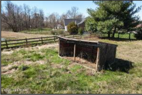
Two animal shelters are well-positioned within the fenced pasture areas
