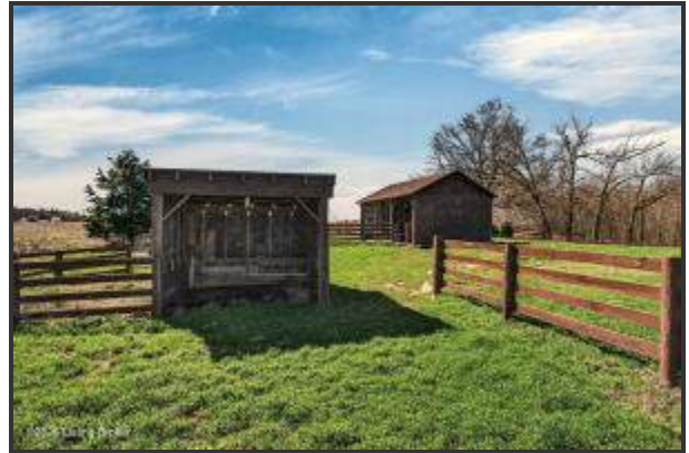
Multiple outbuildings dot the property, adding versatility and function
