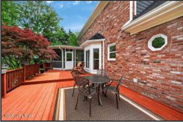
Rich stained wood decking and railings are in excellent condition throughout
