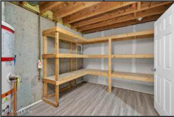
Lower Level: Utility Room
