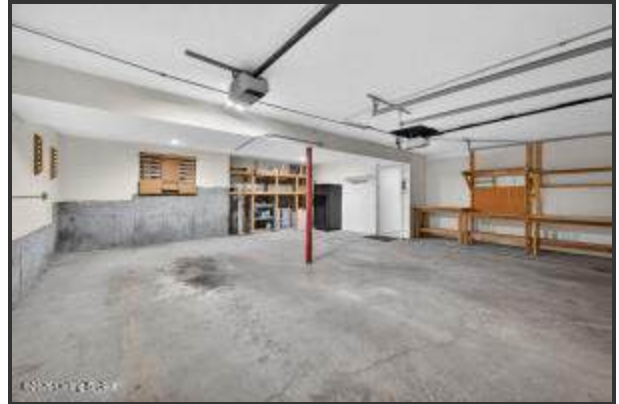
A built-in workbench and shelving offer plenty of space for tools and storage in the garage
