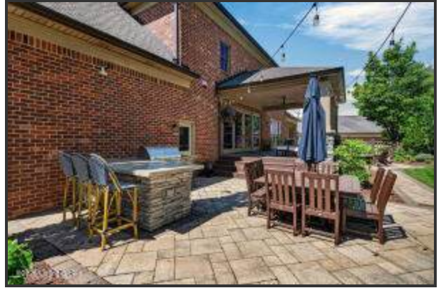
Breakers are already in place for an outdoor hot tub
